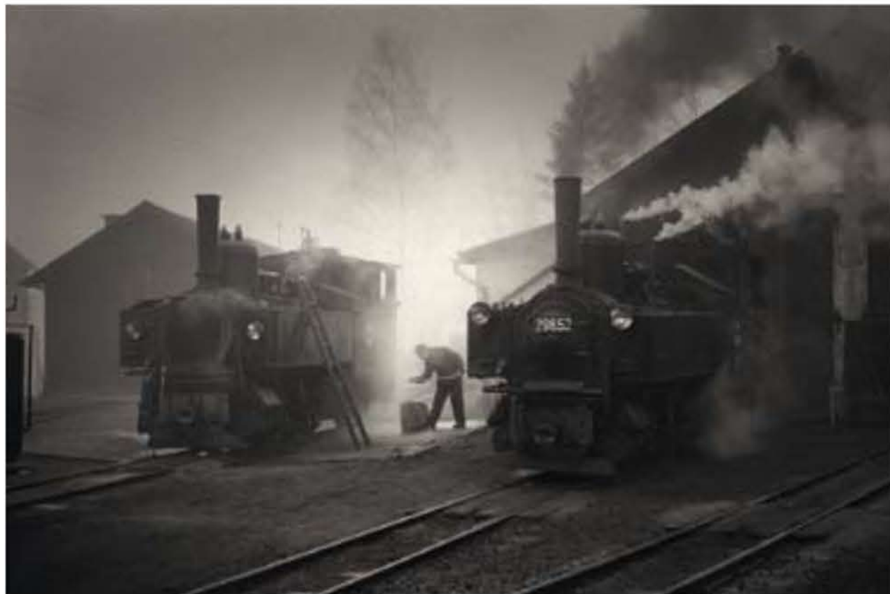
298.53 & 298.52, Heizhaus Garsten, Steyrtal, 1975
